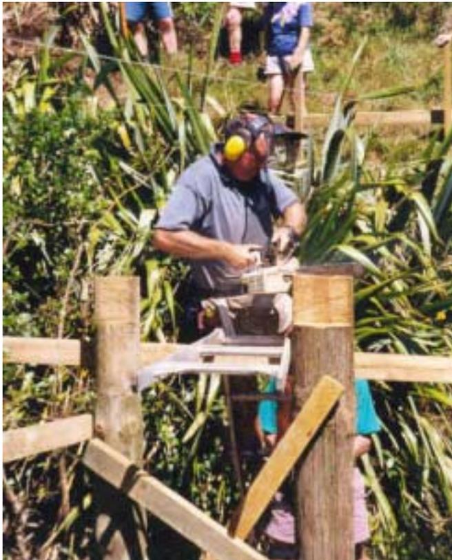
beams. Under the careful supervision of almost-live-in chippie Ian Higgins, we first erected the six posts – two at each end, and two in the middle. A few bags of ready-mix concrete secured them in place, while the main beams were put up. Meanwhile, a gang of six of us hacked and slashed out a new length of track through the wild and dense flax and gorse jungle. (Think I'm exaggerating? Ever tried removing flax in a confined space??)
